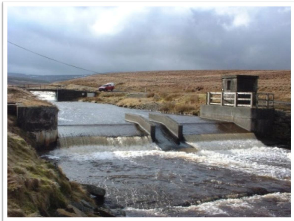
20 – The Trout Beck Gauging Station. This was established in the 1960s but recording ceased in 1979. It was reinstated by the Environmental Change Network in 1991 and since then the Environment Agency have undertaken a major reconstruction. Discharge data are vital for understanding the chemical and biological data gathered from the Trout Beck by ECN. Photo: John Adamson.
